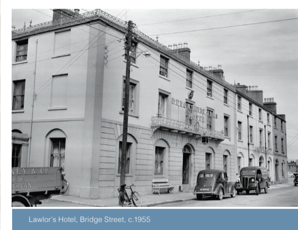
Lawlor's Hotel, Bridge Street, c.1955
